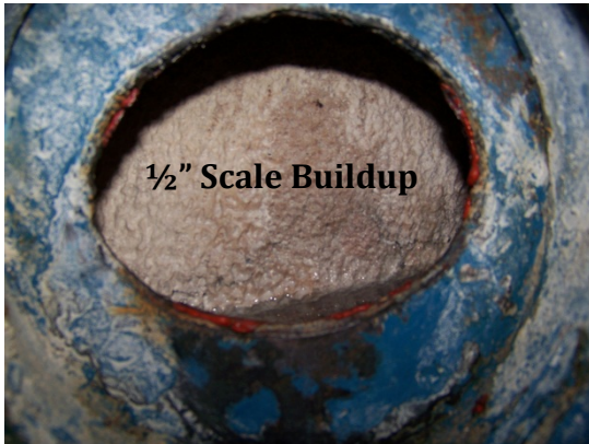
Boiler #1: Bottom Hand Hole before Scale Removal
