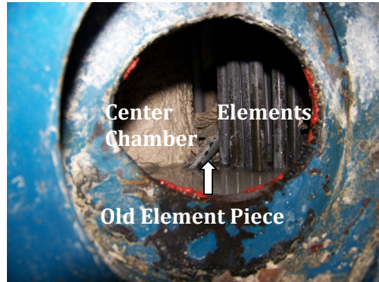
Boiler #1: Bottom Hand Hole after Scale Removal
